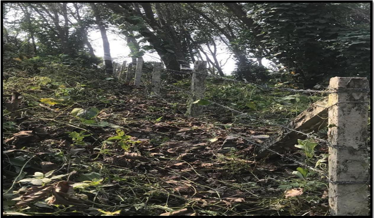
Photograph of Fencing around lease area
