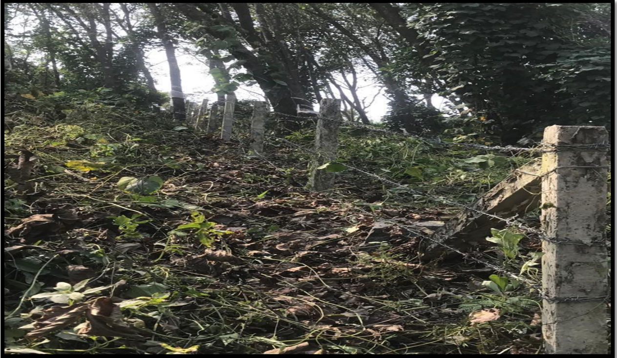
Photograph of Fencing around lease area
