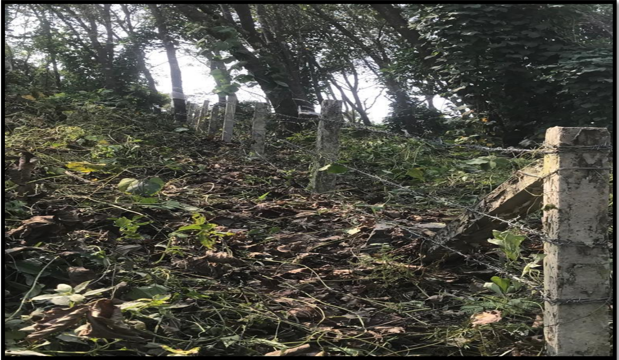
Photograph of Fencing around lease area
